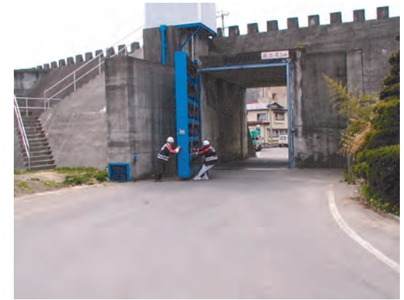
写真⑧消防団員によって閉じられる防浪堤の門 Photo 8: The dike gate closed by firemen
