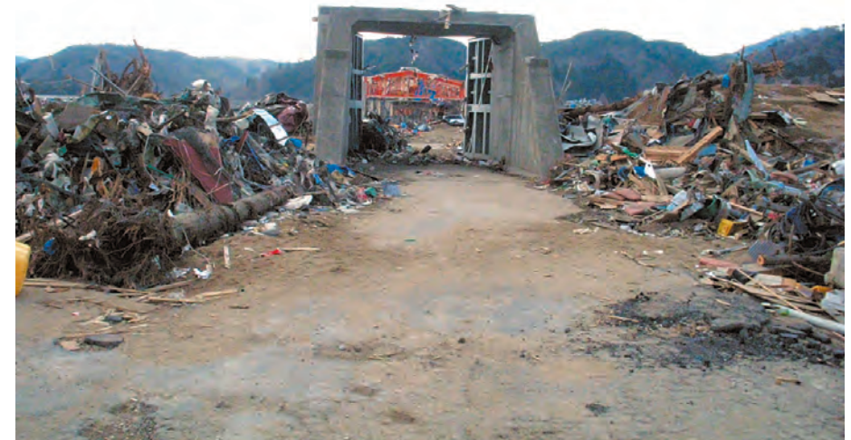
写真⑮防潮堤の門：残ったのは防潮堤の門の枠だけ Photo 15: Only the frame of the gate was left.
